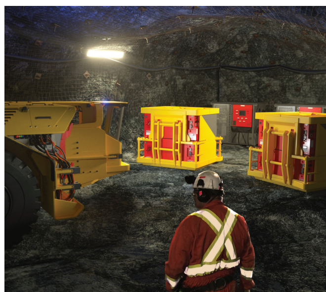
Electric underground equipment at Macassa mine. Image courtesy of Kirkland Lake Gold.
