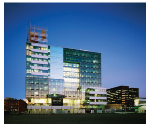
Photo credit: Peter Vandewalker
