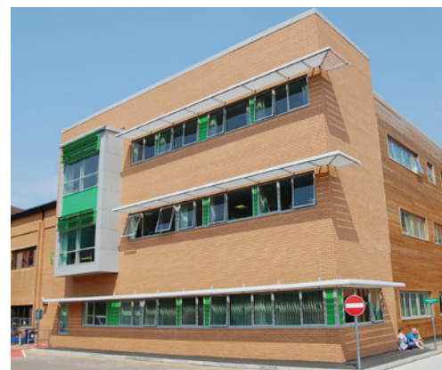
Retrofit designed for life cycle performance: Musgrove Park Hospital, UK
