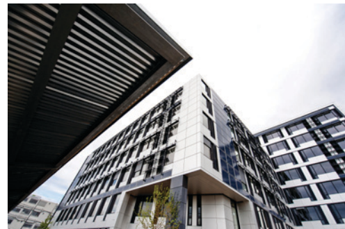
The world's largest positive energy building: Green Office® Meudon, France
